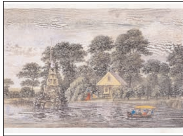
No.4: Fountain Cottage, Camberwell, c. 1794
