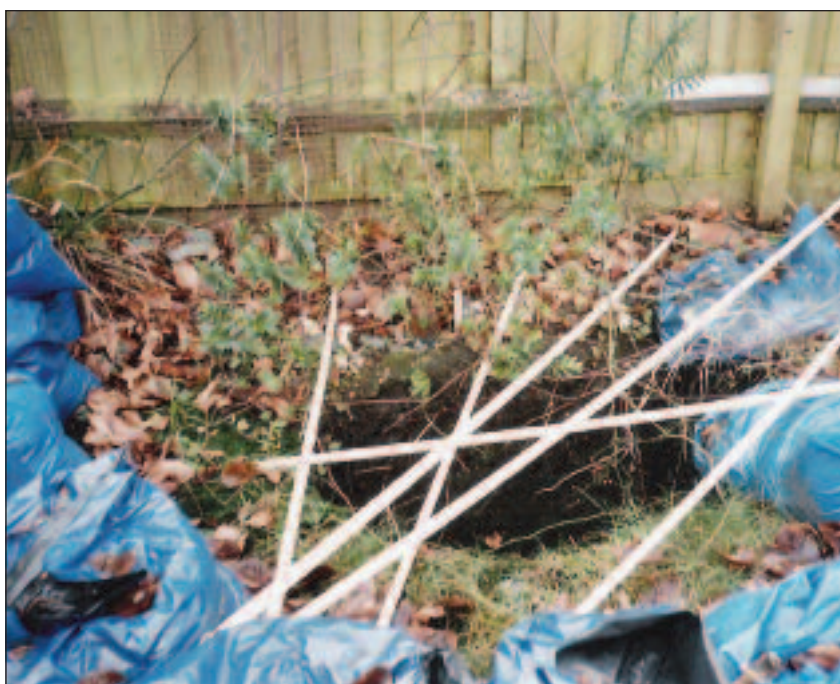
Look into the hole and you can see the old brickwork belonging to the well
