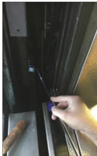
Checking a lift shaft
